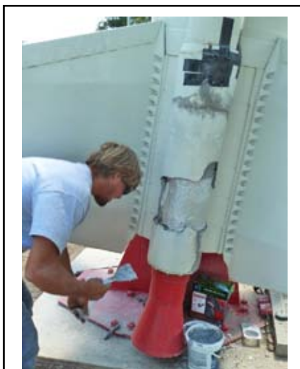
John Henry making Athena repairs. Courtesy photo.
