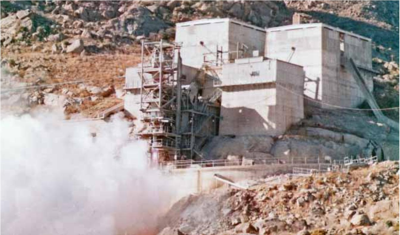
**A Redstone motor under test at the 500K Static Test Stand. As you drive along War Road and look at 500K, it appears there is a tunnel below the stand. That is an area that has been hollowed out by the super hot exhaust gases from the tests hitting the granite and then the spray of water from above to cool everything. Yards of rock have spalled off the face over the years creating an alcove under the facility. Courtesy photo**
